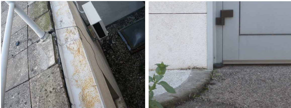
Fig. 14. STER PMU installation – typical location for the GPS antenna
