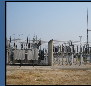
TE-TO Zagreb, during installation
