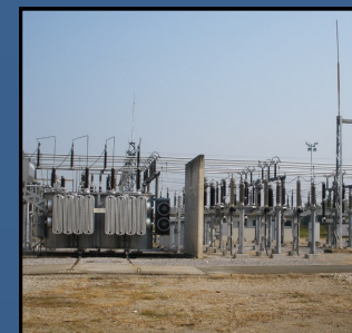
TE-TO Zagreb, during installation
